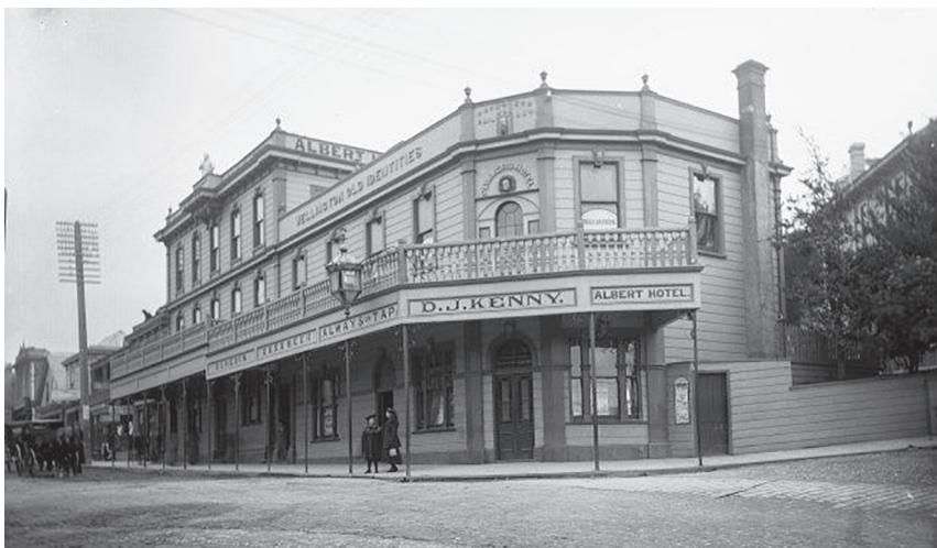
Early photograph of the Albert Hotel, Willis Street, Wellington. Note telephone wires are evident but no motor cars, at least in this pic. Acknowledgement: National Library of NZ website.
