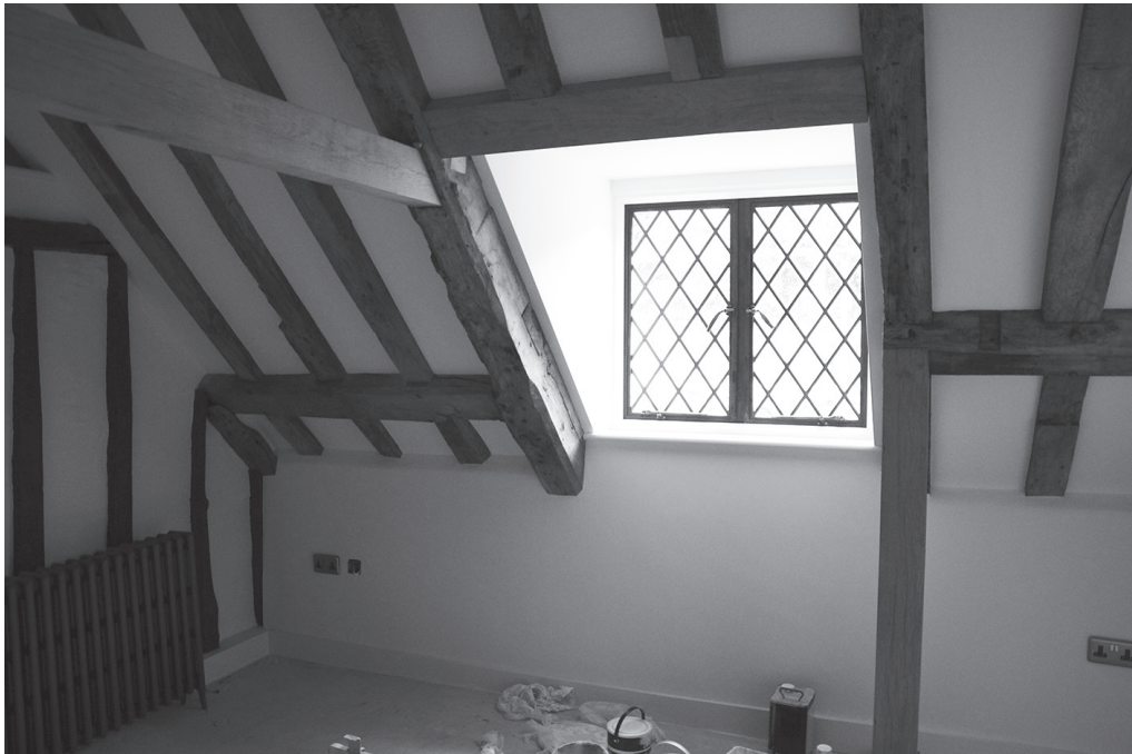
Attic room with oak beams exposed.
