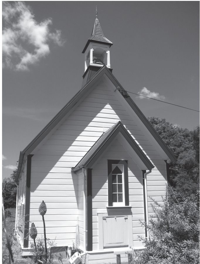
St Aidan's church, porch-end view, showing narrow width of the building (designed for a congregation of 50). Note the small door set low — which allows passage of coffins. Normal passage of coffins was not possible owing to the 'tight turn' between nave and porch door.
