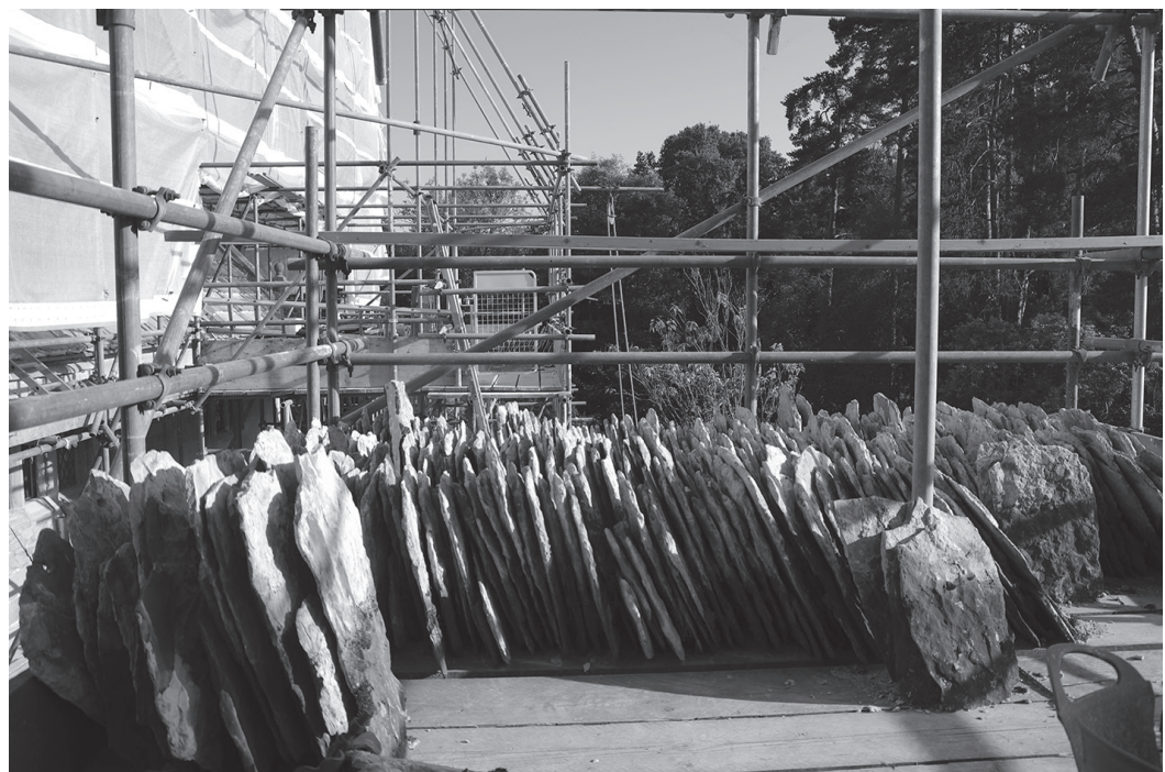
Horsham stone roof tiles stacked on scaffolding, ready for re-laying.
