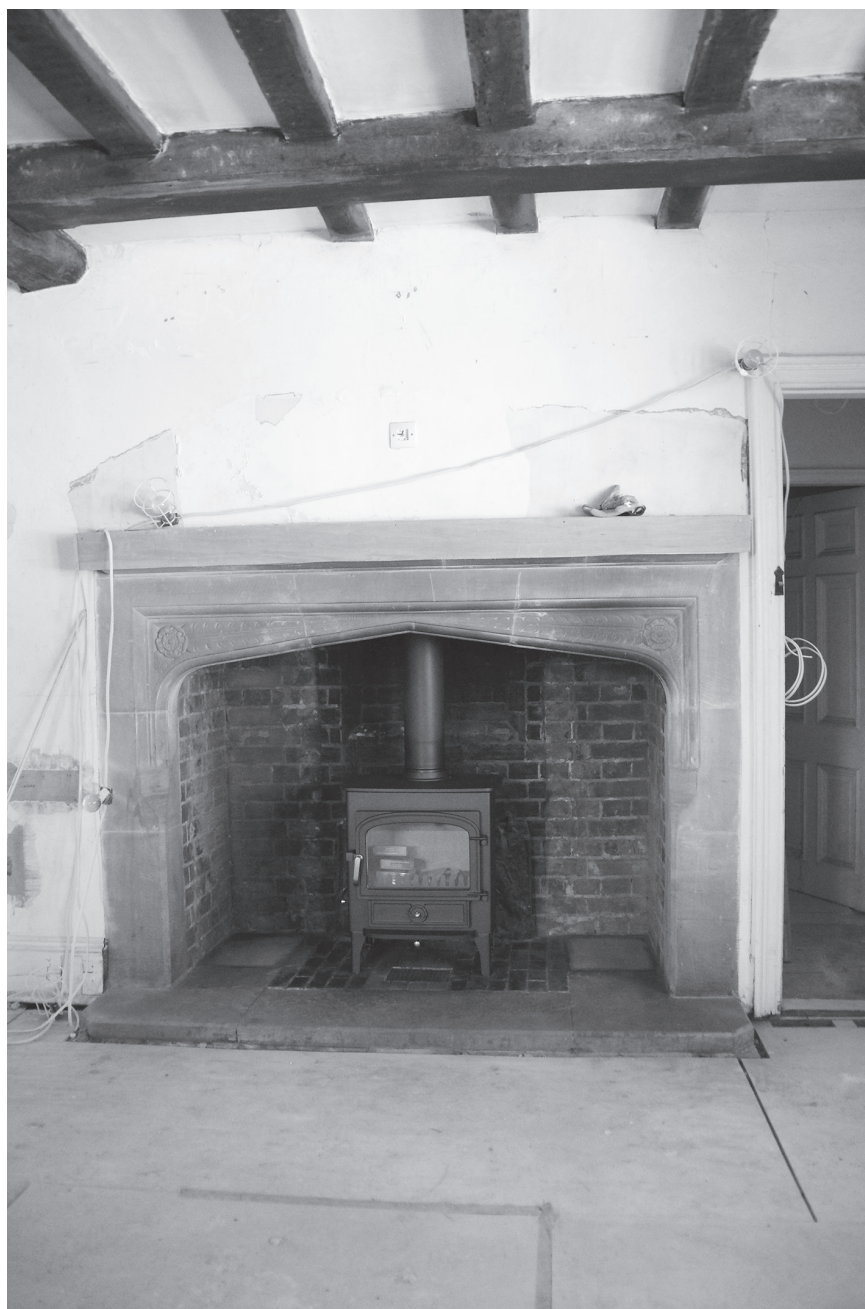
Fireplace restored to original size with wood burner installed.
