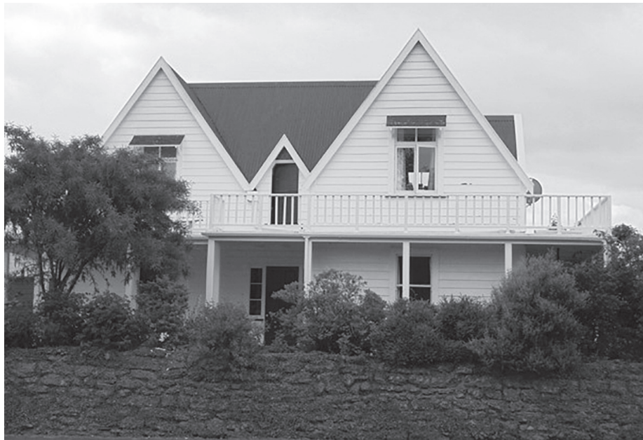
The Field family home was built of heart Kauri timbers (1868). It is located on Field's Track, between Kakatahi on the Parapara road and Karioi, near Tangawai.
