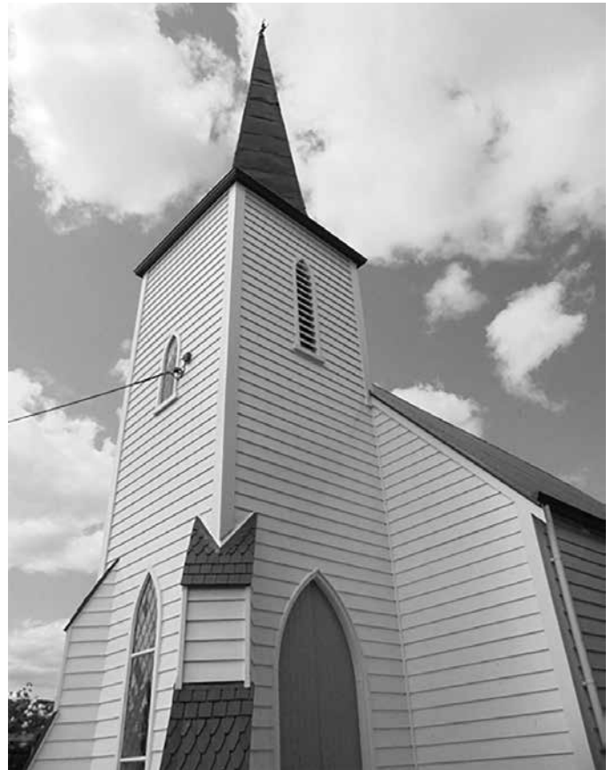
Right: St Mary's church, Upokongaro, note the three-sided spire on a four-sided tower.
