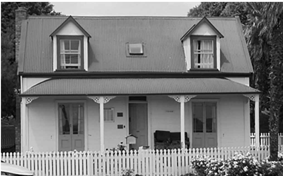
'Tylee cottage,' built 1853, shows features of early cottages, with front verandah, central door and rooms either side.
