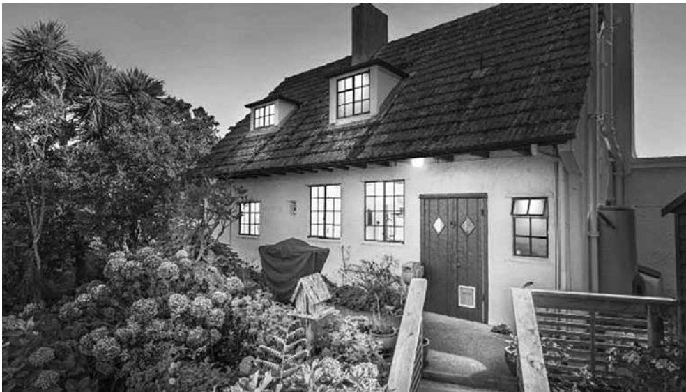
A James Chapman-Taylor-designed cottage in Khandallah, Wellington, built in 1935. Signature features of his style included concrete walls, a tiled roof and interiors that featured an 'arts and crafts' look with prominent timbers and joinery.
