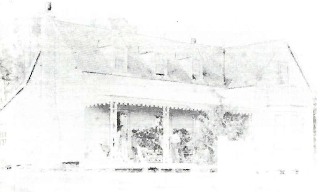
The second Mount Vernon Homestead prior to 1882. Dormer windows and shingle roof were typical of New Zealand colonial architecture of the period.
