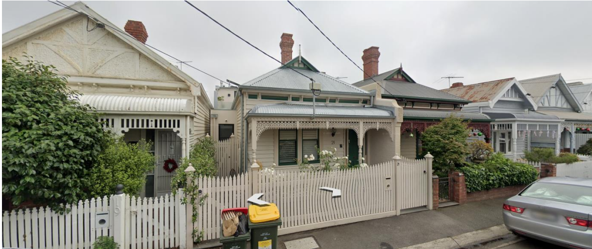
Densely packed cottages along Port Melbourne's Albert st.
