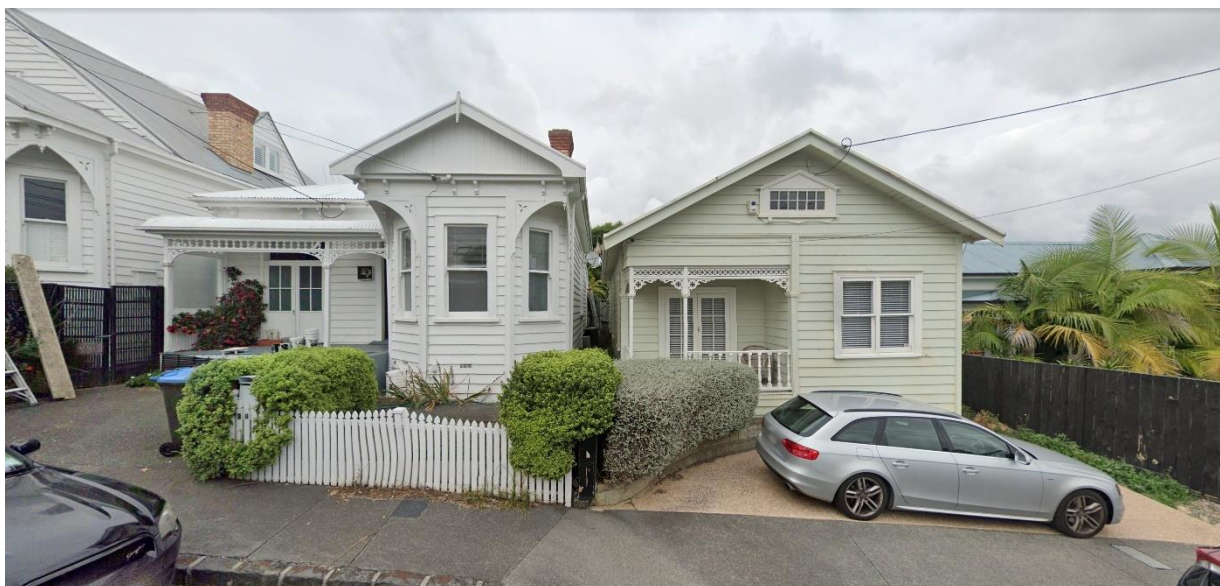
An ornate late Victorian villa (left) next to a transitional villa (right): note the similar spatial articulation below the roofs.
